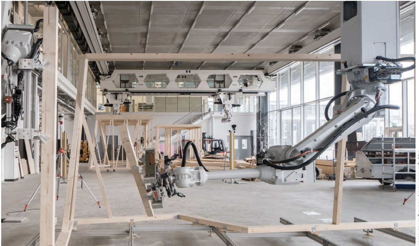
Copyright Roman Keller / NCCR Digital Fabrication.
